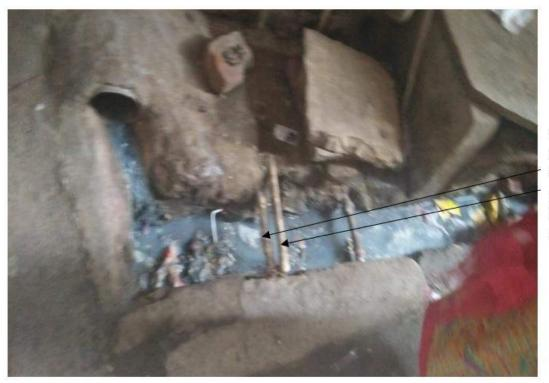
Prone for cross contamination due to overlapping of pipeline and in close proximity of sewage water. This is the common finding in Bhadola village
