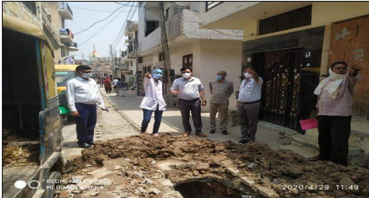
Fig. 5: Identifying leakages in pipelines with PH Department
