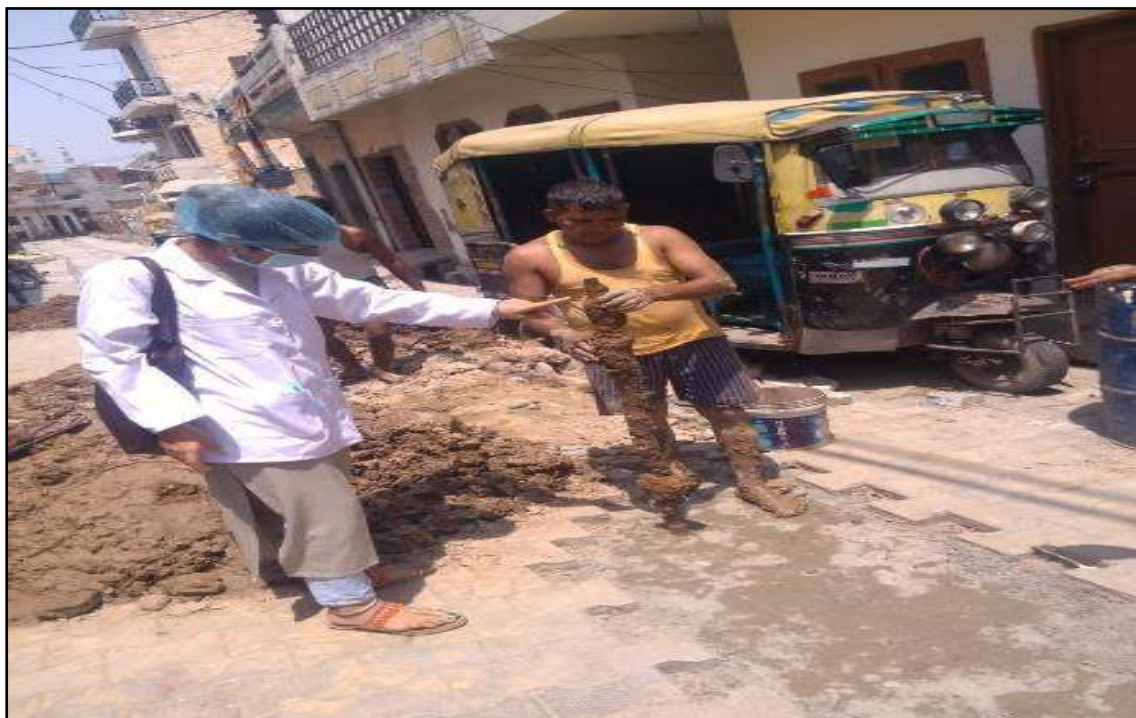
Fig. 6: Removal of leaked and rusted pipelines
