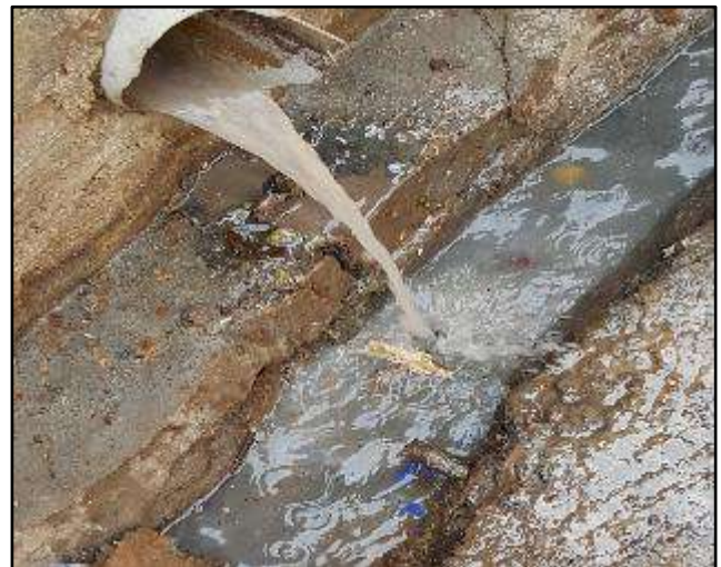
Pic.2: Water pipeline along open drains
