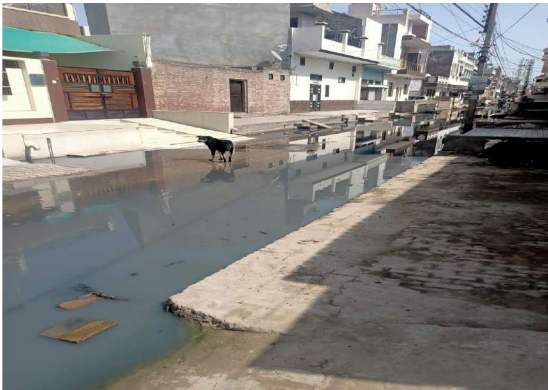
Figure 2: Reverse flow from gutters (Photo 1)
